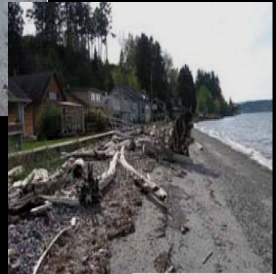
Puget Sound - beach replenishment with buried bulkhead
